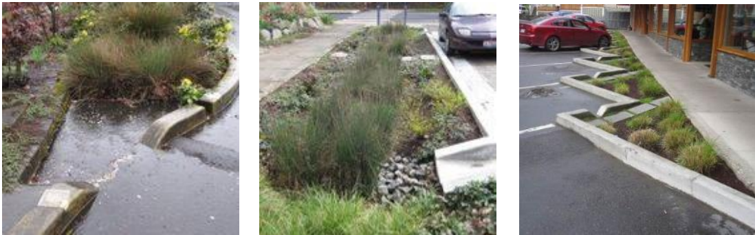
Rain gardens in Toronto taking surface water from car park and pedestrian areas (Photos: Dusty Gedge).
