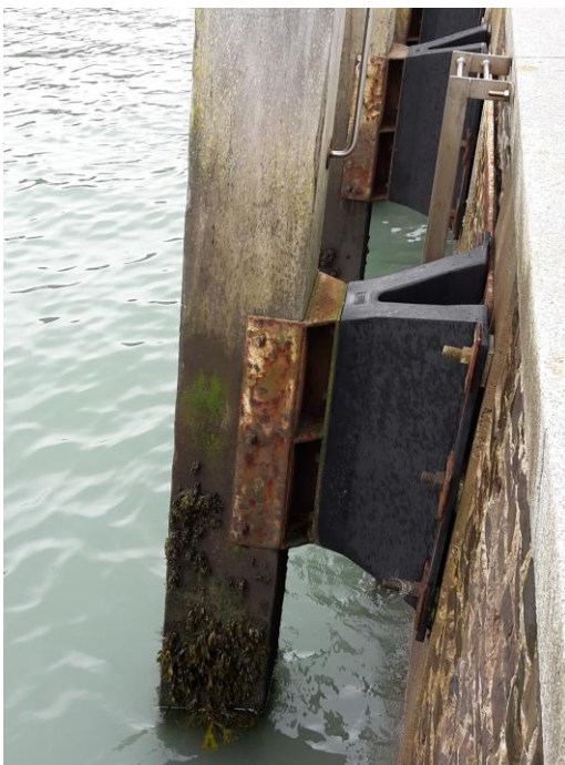
Timber baulking attached to dock using rubber shoes © Ben Kimpton.
