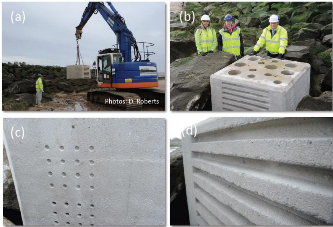
Figure S5. The BIOBLOCK at Colwyn Bay, Wales. (a) The unit being lifted into place by a crane; (b) top-down view of unit showing scale and the three faces with multiple habitat types; (c) areas (25 x 25 cm) with pits that are either shallow (2 cm, top) or deep (5 cm, bottom); (d) sidelong view showing longitudinal horizontal crevices.
