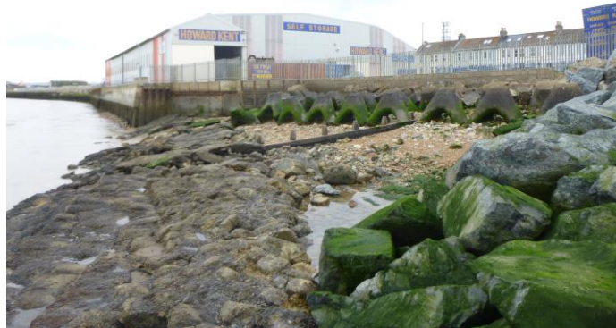
Shingle, mixed artificial substrates and rock armour revetment at the beach adjacent to RNL Shoreham Lifeboat Station. Forms the eastern end of SS4 © TEC.
